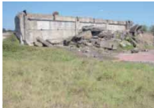
Figure 13: Ruin of the Former Williamstown Racecourse Grandstand at Altona Coastal Park
