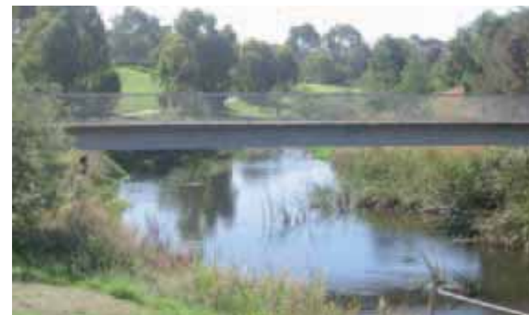
Figure 7: Footbridge over Kororoit Creek at the end of Billingham Road in Deer Park
